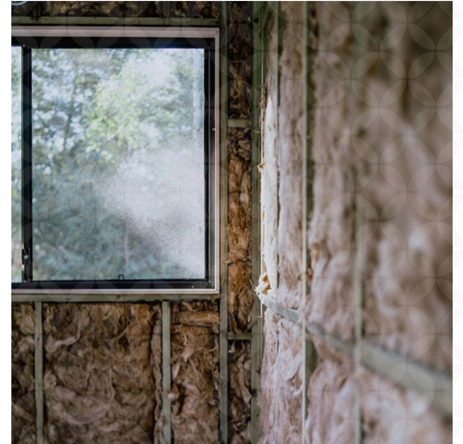
◆ FIGURE 11 Insulation in stud walls SOURCE: Earthwool
